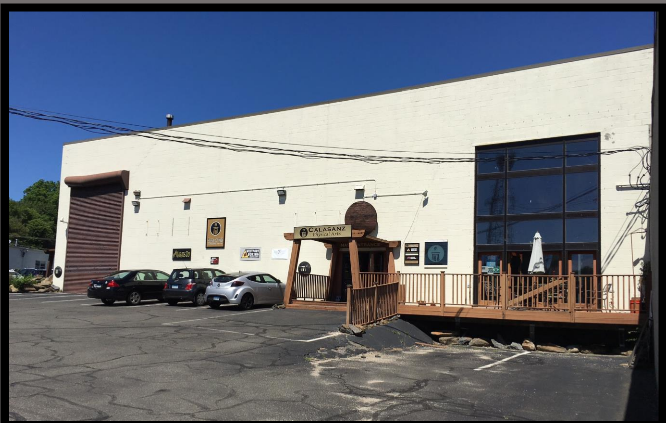
Rear Portion of Building
