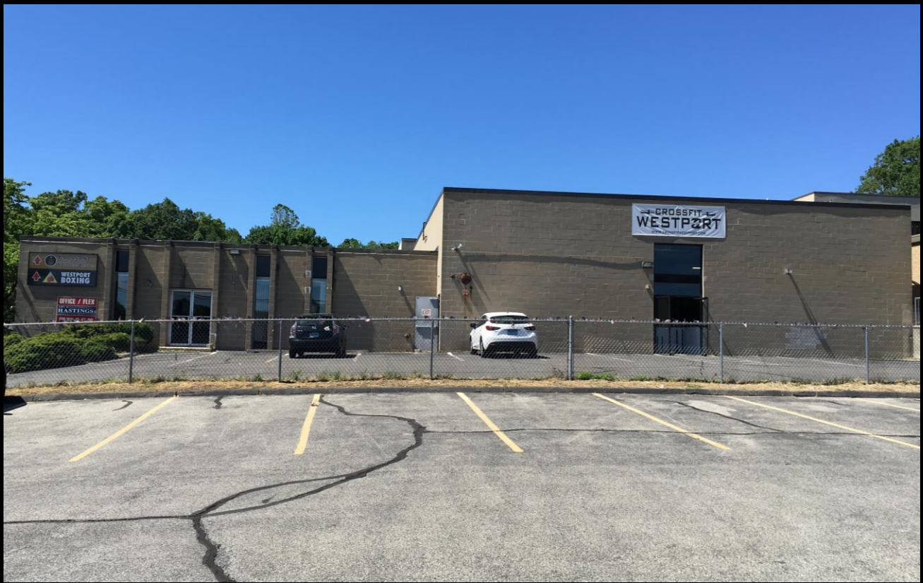
Front Portion of Building
