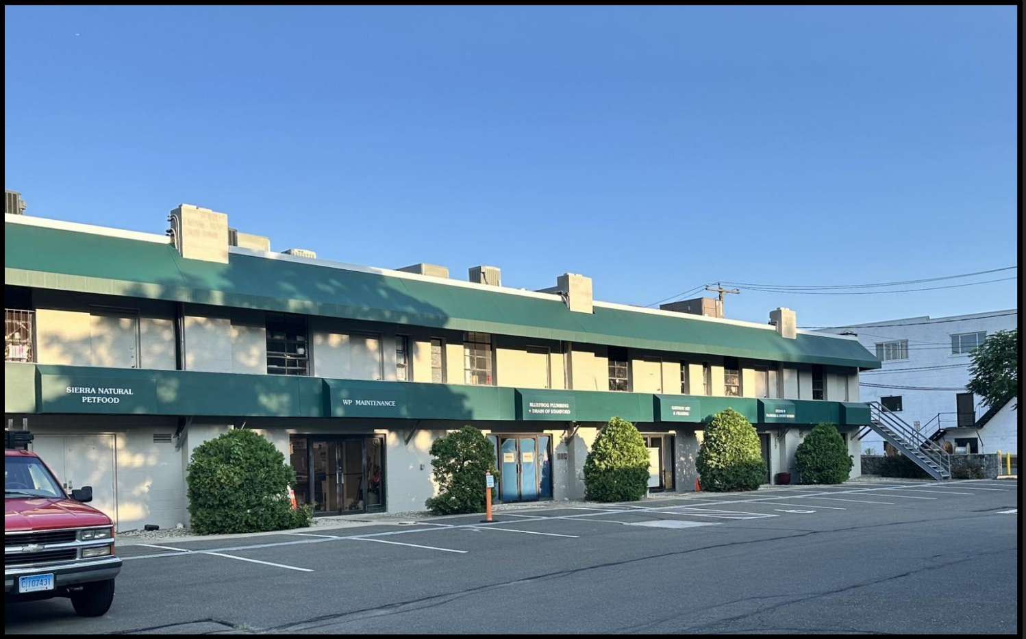
North & South Views of Rear Parking Area/Available Space
